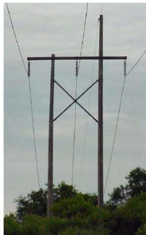
Figure 2.1-1 Conventional 115-kV line with 3650mm phase-phase spacing.
